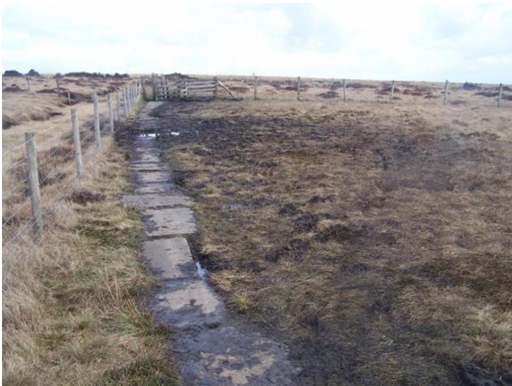
Damage to vegetation caused by one missing flag in the footpath, summit of Winter Hill (26 March 2014)
