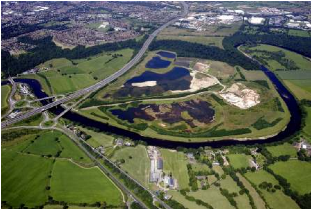
Fig 1 The Brockholes Site and the M6 Looking North
